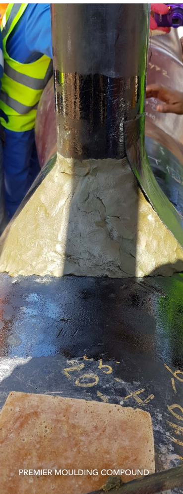
Section of pipe with Premtape LD Mastic applied
