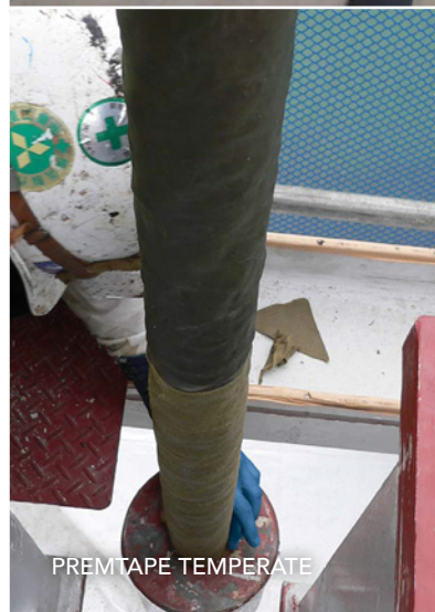
MACALLOY BARS PROTECTED WITH THE THREE-PART SYSTEM
