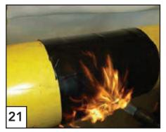
Beginning below, heat the middle of the sleeve, moving the torch in a circumferential direction with blue-yellow flame. Use the same motion to shrink one side, then the other side. Ensure even shrinkage.
