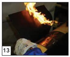
Wrap the sleeve around the pipe tightly. Position it carefully and warm up the butyl rubber with a blue-yellow flame.
