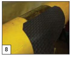
Place the sleeve on the preheated area of the pipe.
