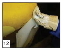
Remove the release film completely from the remainder of the sleeve.
