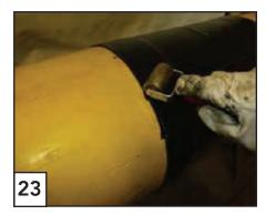
Roller the transition to the factory coating, the edge of the sleeve, the overlap of the sleeve and the area of the welded seam.
