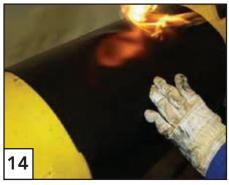
Stick the sleeve all the way around the pipe overlapping onto the underlap. Warm the overlapping area.
