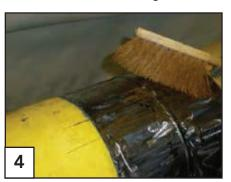
The surface of the steel and adjacent coating shall be free from grease, oil, and dust. If solvent cleaning is required this shall be carried out according to Steel Structure Painting Council SSPC SP 1 using approved solvent.
