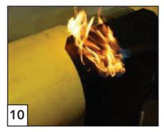
Heat the applied end of the sleeve with a blue-yellow flame, so that a 20 cm portion of the sleeve sticks to the pipe.
