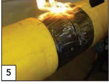
Dry the pipe and warm the area where the sleeve will overlap itself (exposed pipe plus adjacent factory coating) to 50°C.
