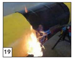
Continue warming the adhesive side of the closure patch and position it over the whole sleeve width in the overlapping area.
