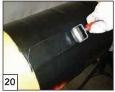
Roller the closure patch in the overlapping area. Let the installed closure patch cool down before continuing with application.
