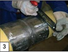
Abrade the adjacent factory coating (including the beveled edges) 100 mm on both sides of the joint.
