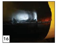
A bead of extruded butyl rubber is visible at the edge of the sleeve.
