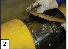
Preheat the pipe to remove moisture, if necessary. Clean the pipe surface thouroughly to very thouroughly (St 2 - St 3) with a hand wire brush. Remove rust, dirt and other residues.
