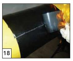
Progressively warm along the length of the closure patch and press it on until butyl adhesive is visible out of the side.
