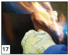
Warm one end of the adhesive side of the closure patch with a gas flame. Position the warmed side of the closure patch over the exposed edge of the sleeve.
