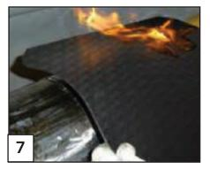
Remove approx 300 mm of the release film from the whole width of the mitred end of the sleeve. Warm up the butyl rubber using the Propane torch.
