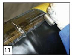
Roll on the edges of the end of the sleeve with a roller until butyl rubber flows out of the sides.
