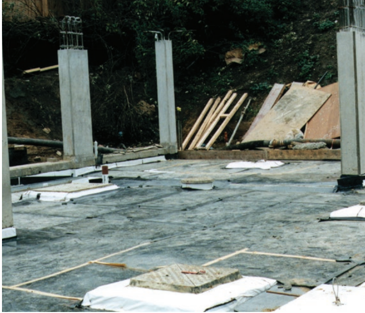
Premseal GMA™ used on new foundations in the construction of an apartment block.
