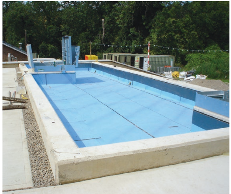
Premseal 100™ used in a tanking application.
